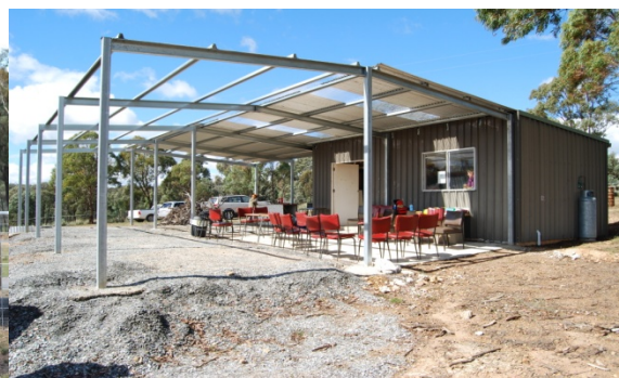
The clubhouse extension
